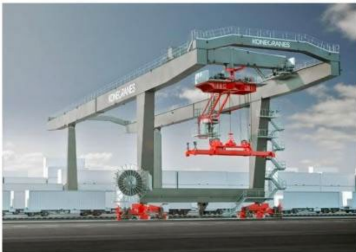
Figure 4: Rail-mounted Gantry crane
